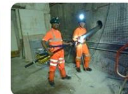
Bore hole detector installation
