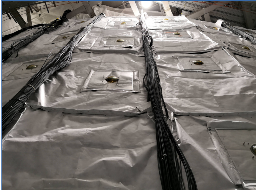
Tyvek installation in Super-Kamiokande [3]
