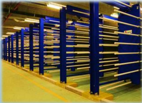
Heat exchangers on Toronto’s City Potable Water Network (2006) (400'000 m 3 /day, 4 °C => 12 °C)
