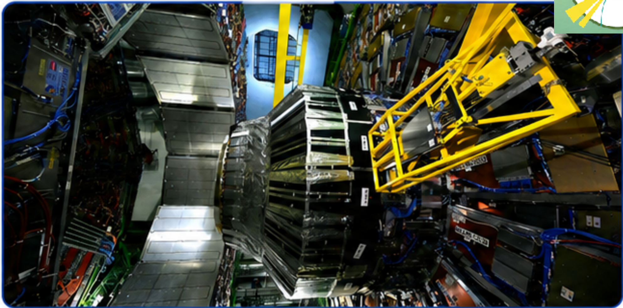
Representative CMS GE1/1 GEM installation.
