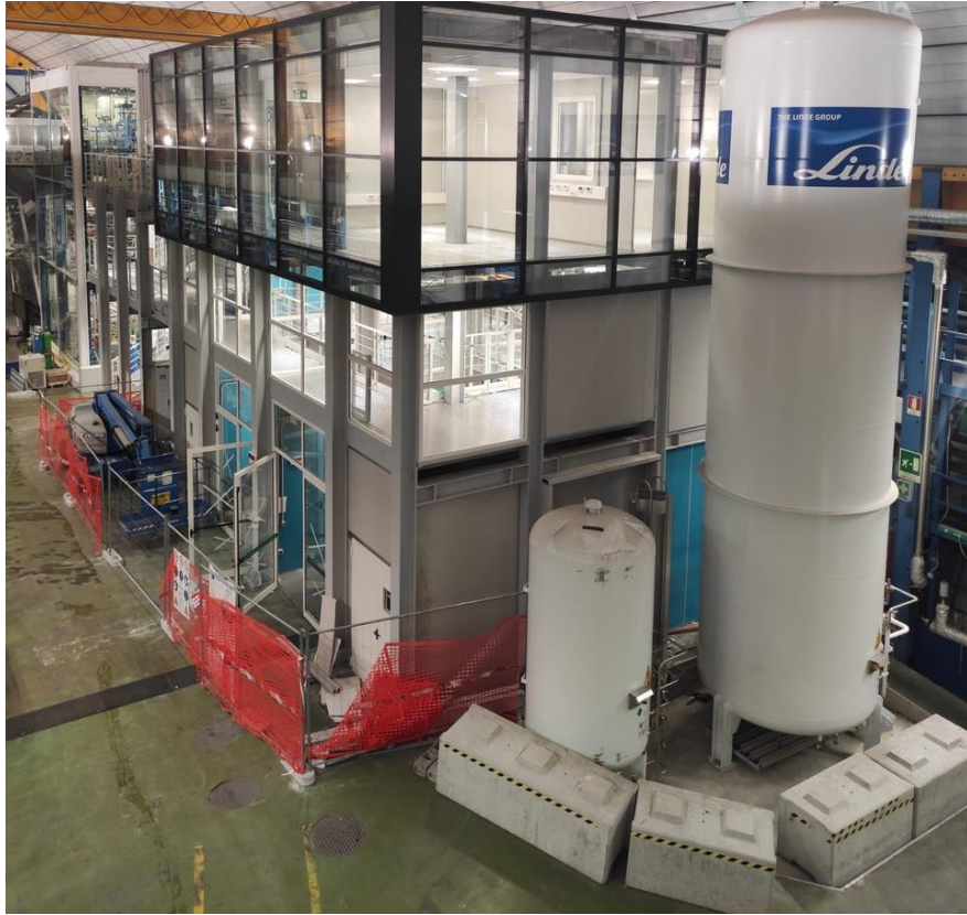
Cryoplatfrom, Hall B, LNGS – under construction
