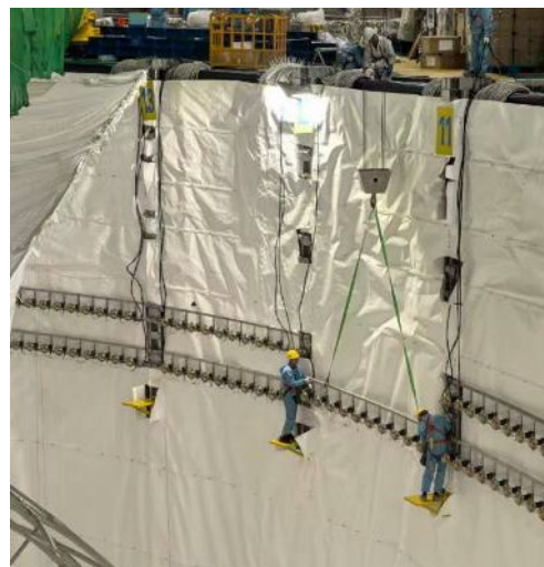
PMT and Underwater box installation
