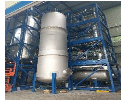
2) Distillation for radiopurity
