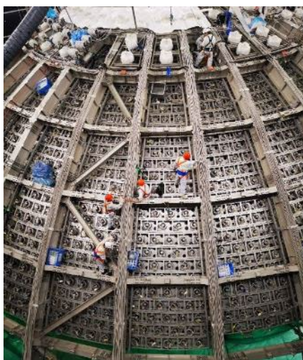
PMT and Underwater box installation
