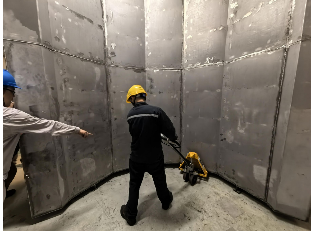
Water tanks positioning around CD tank
