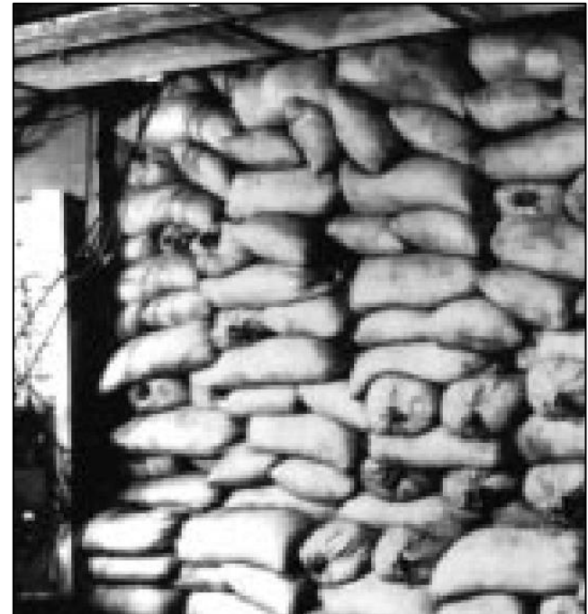
Wet sawdust shielding
