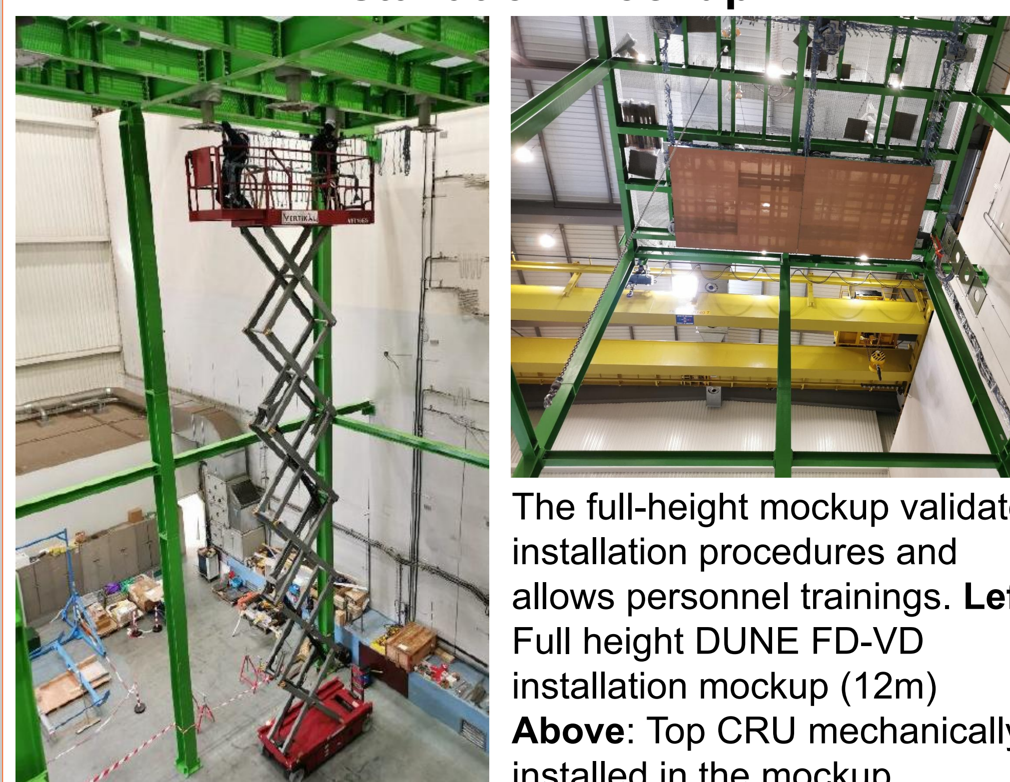
Bottom CRP installation requires CRU rotation. Installation tooling and flip procedures were validated at CERN in 2025.
