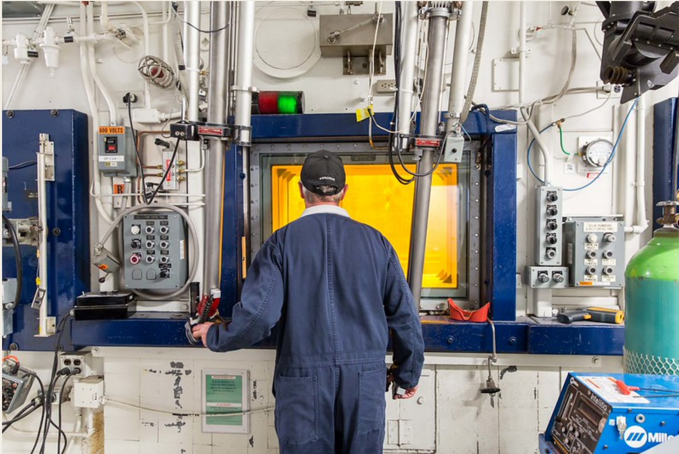
Hot cell at CNL
