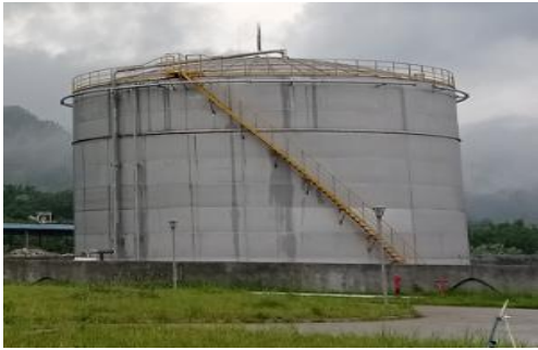
5000 m 3 LAB storage tank
