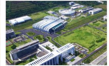
China Spallation Neutron Source (CSNS)
