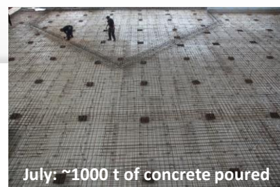
July: ~1000 t of concrete poured
