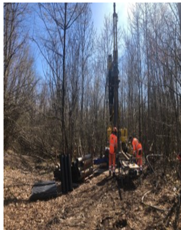
(b) Works started
