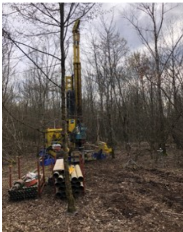
(a) Drilling machine in place
