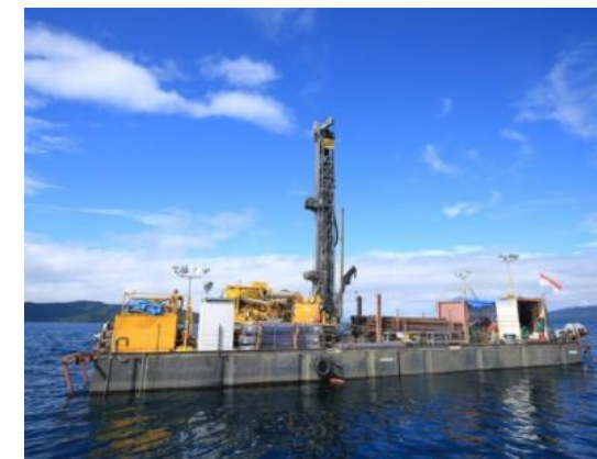
Drilling works on the lake
