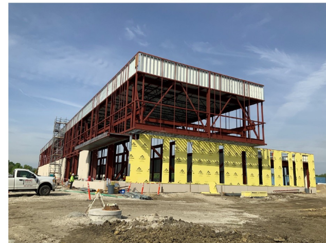
PIP-II construction May 2022
